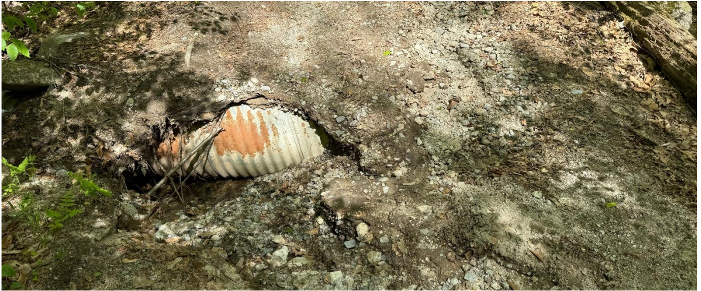
Newly eroded culvert 2025
