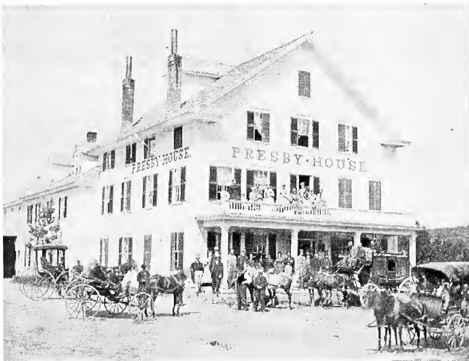
The Presby house was destroyed by fire October 12 1873. The Brown Memorial Library now occupies the site.
